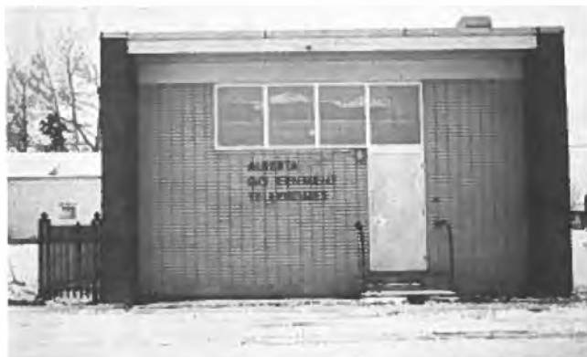
Andrew Telephone Exchange Building.
