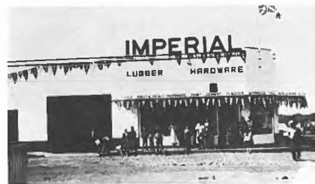
Official opening of the present Imperial Lumber Co. building.
