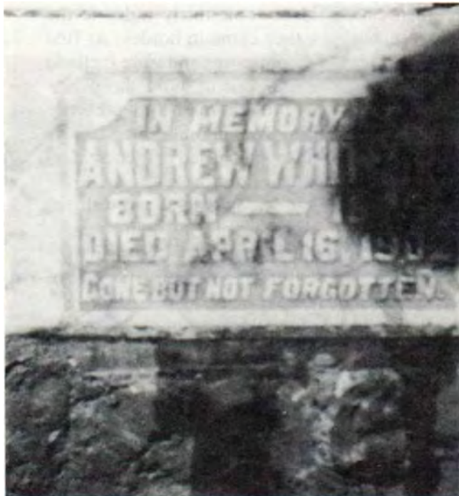
Memorial stone used as the cornerstone in the Village office.
