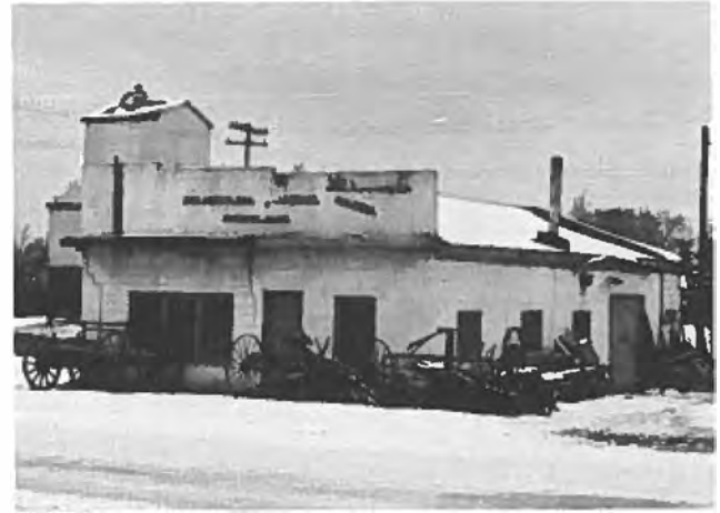
J. Frunchak's welding shop.
