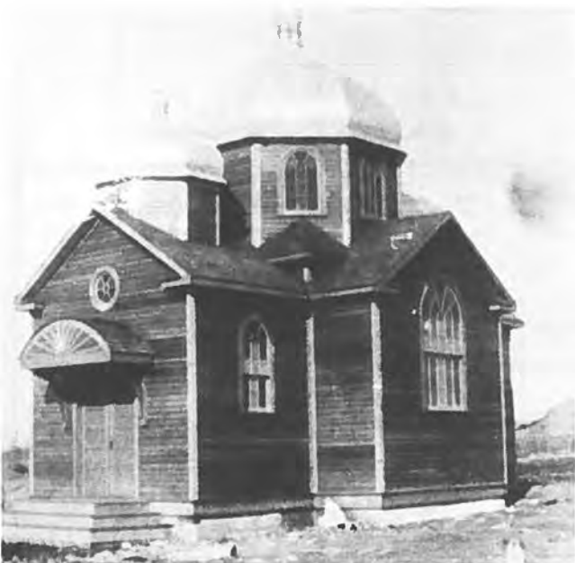
Zawale Church under construction in spring of 1930.
