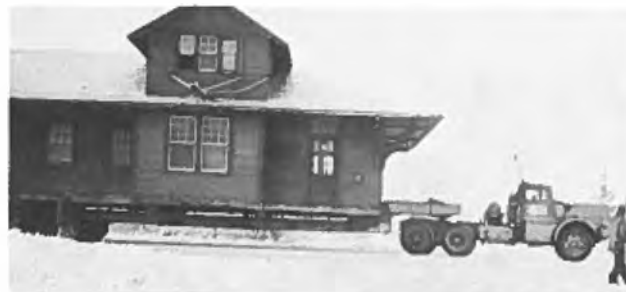
Zidar Brothers moving the C.P.R. station to a new location to serve as the Andrew Museum.
