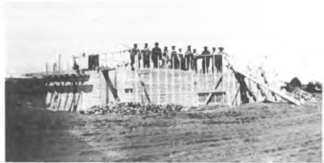
Construction of Kysylew Church, 1950.
