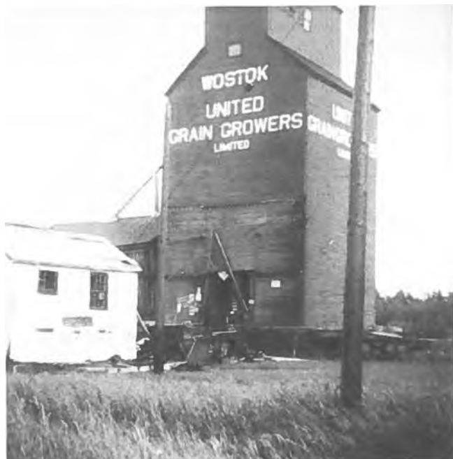
Damage done by the tornado on June 23, 1971.
