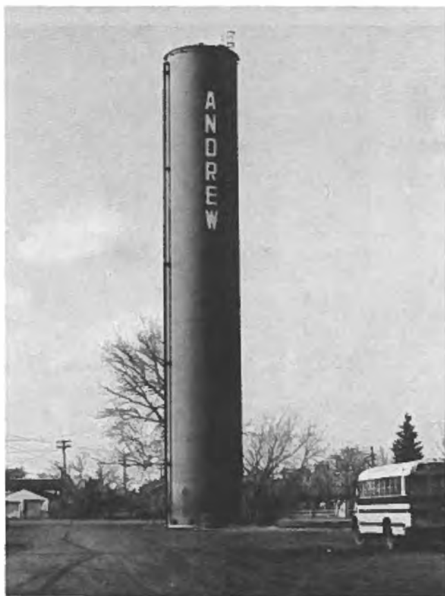
Andrew landmark — water reservoir.
