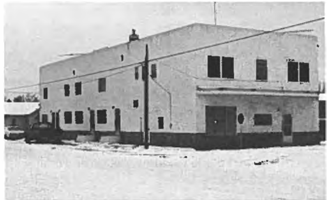
Roxella Theatre remodelled into an apartment building.
