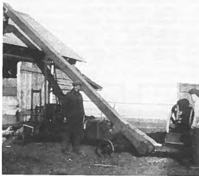
Wooden grain elevator on Hudema farm.
