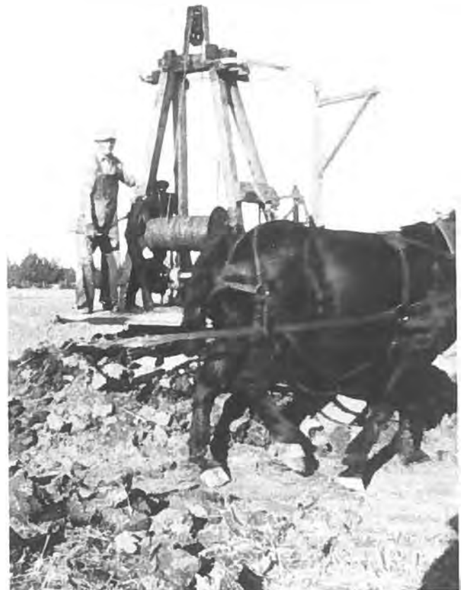
Alex Woychuk drilling wells.
