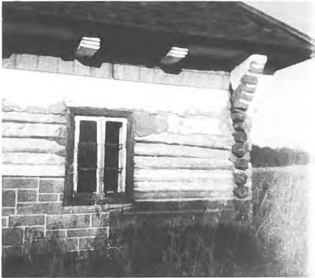
Note the design in the ceiling joists.
