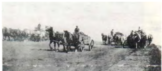
Construction of the railroad bed, 1928.
