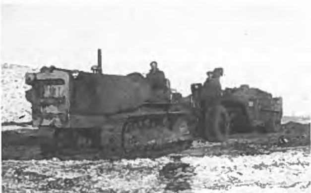
Eagle Construction — building roads.
